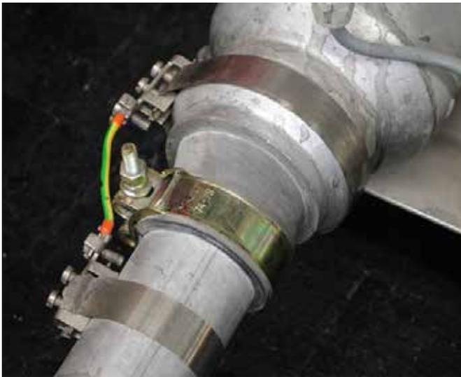
**Figure 25** Ground connection on pipe system
